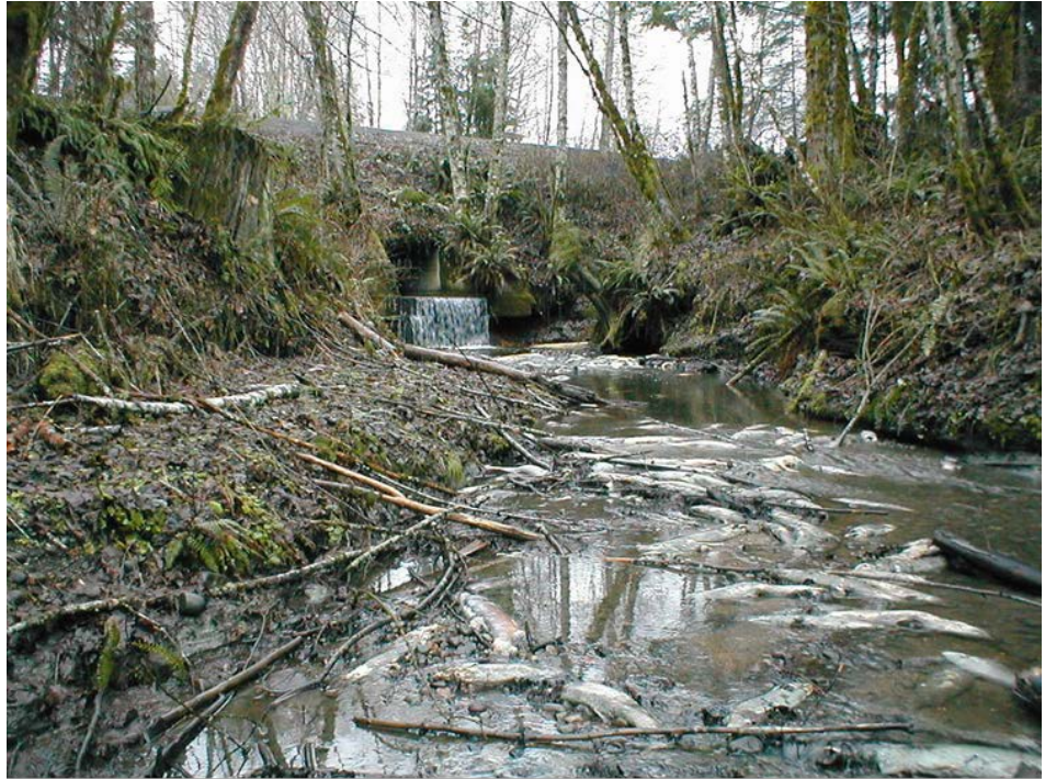
Carcasses of coho salmon blocked by a barrier culvert. Photo credit: WDFW
