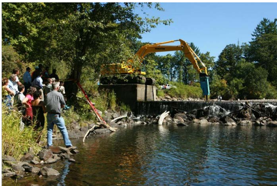
Brownsville Dam Removal, Oregon. Photo credit: NOAA
