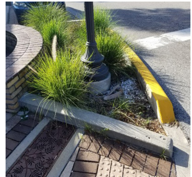
Figure 22. Green infrastructure like this rain garden with curb cut is an example of Accommodation. Low impact development and Green infrastructure in upstream locations reduce downstream flows by allowing more stormwater to infiltrate in place, thereby taking the pressure off the existing downstream stormwater infrastructure. Photo by Atkins, 5th Street, Palmetto, Florida.
