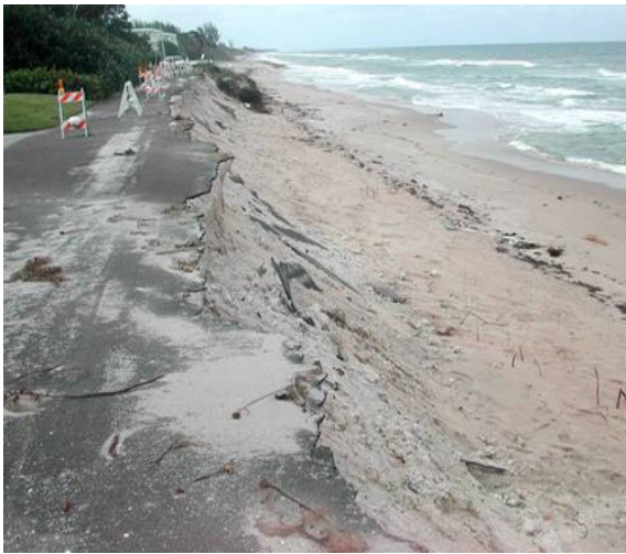
Photos (above): Road erosion on Old South Ocean Boulevard due to Hurricane Frances in 2004 in Palm Beach County, Florida (before and after). Courtesy of the Palm Beach County Department of Environmental Resources Management (2004).
